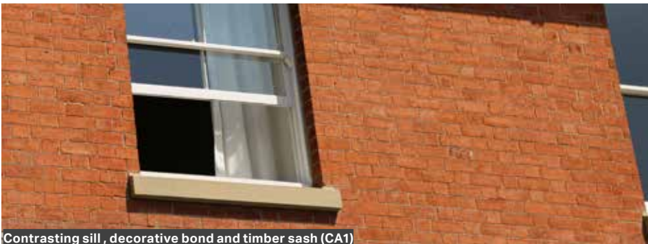
Contrasting sill, decorative bond and timber sash (CA1)
