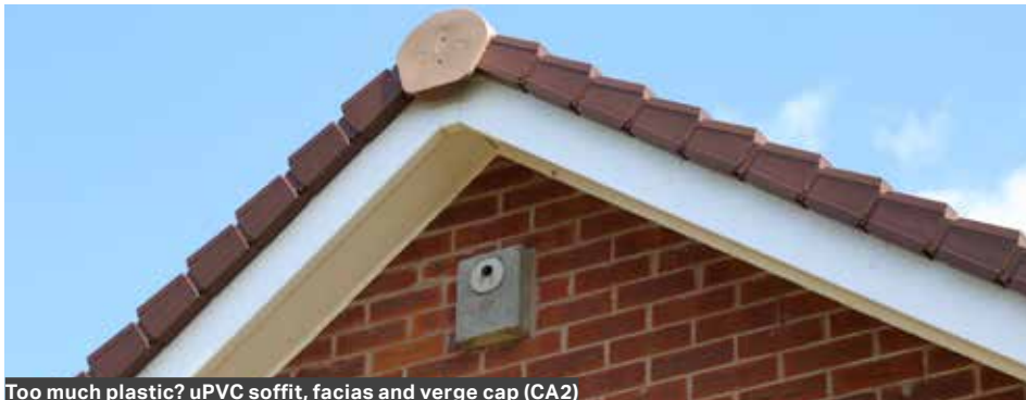
Too much plastic? uPVC soffit, fascias and verge cap (CA2)
